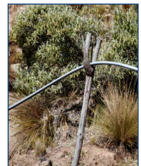
Existing Pipe Support
